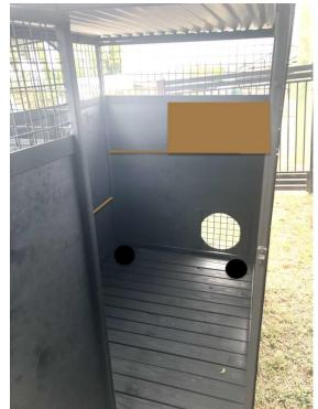
Figure 1: Inside view of prototype Vennel showing roof, ventilation mesh at the top of the wall, shelf and nest box, hole in the wall where the Tasmanian devil PVC pipe trap would be attached on the outside, and holes in the wooden floor for removal of faeces. This design has been modified, and the Vennel is bigger with an insulated overhanging roof and walls made from insulation panels used for cool rooms.
